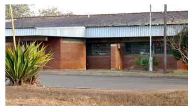
CVL main building which houses the vaccine production unit and other diagnostic and post-mortem rooms
